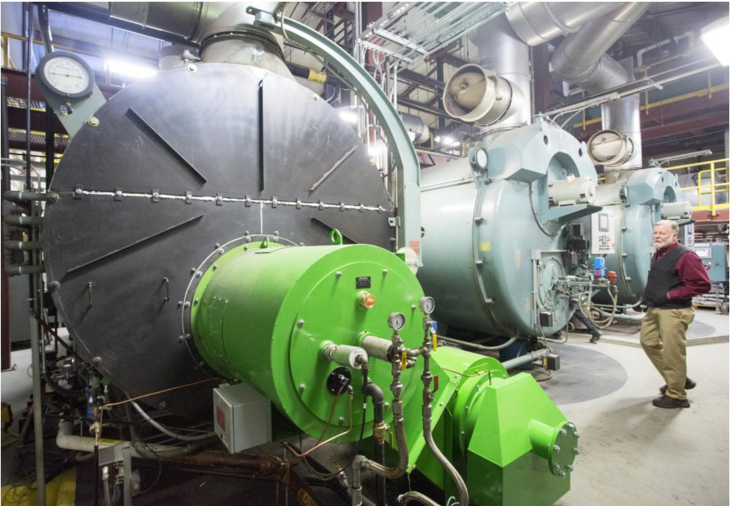
Bates College energy manager John Rasmussen gives a tour of the boiler room housing a new unit, left, that burns wood waste-derived biofuel from Ensyn Corp. The school switched to the new fuel in January to reduce its carbon footprint, and Rasmussen expects the investment to pay for itself within five years. Staff photo by Derek Davis
