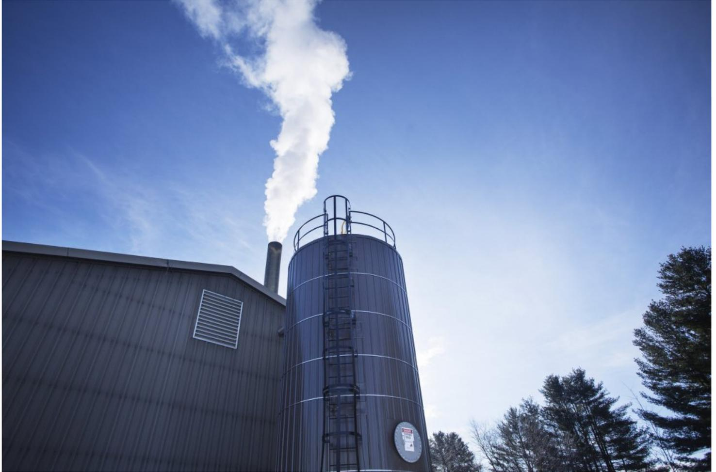
Boiler exhaust rises from a smokestack at Bates College in Lewiston. The school is using wood-derived fuel from Ensyn Corp. in Canada to heat 70 percent of campus buildings. Delivery trucks fill its 20,000-gallon fuel tank five or six times a week. Staff photo by Derek Davis
