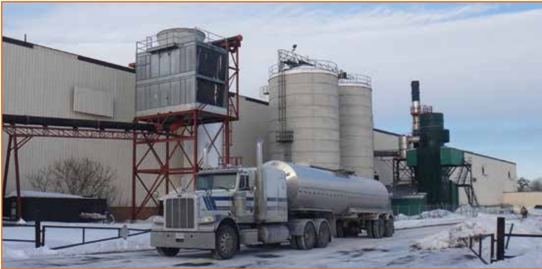
Ensyn's cellulosic biofuel production plant in Renfrew, Ontario
